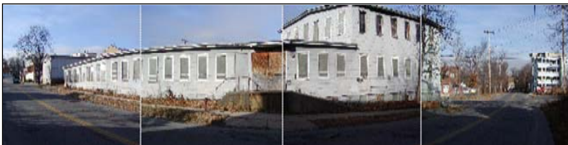
39 SPRUCE STREET (WEST)
